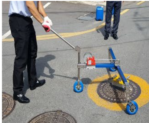
Place the magnet on Manhole center
