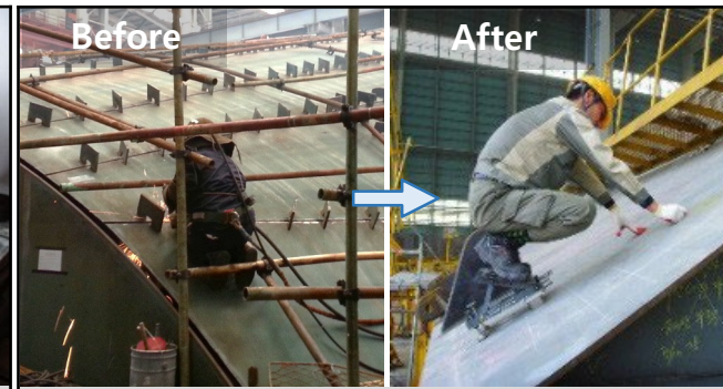
Magnetic Scaffold for Slop works
